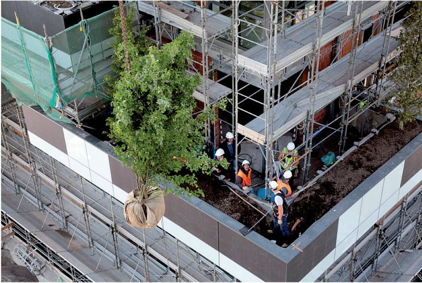
III. 9. Bosco Verticale, Vertical Forest. The steel-reinforced concrete balconies were designed to be 28 cm thick, with 1.30 metre parapets (Image: Boeri)
