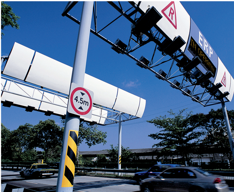
III. 8. The entry into the CBD (Central Business District) zone, Singapore (Source: www.transportpolicy2013.blogspot.ca )
