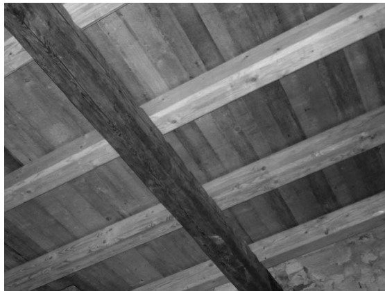
Fig. 5. New and old (recovered) structural elements used as part of the ceilings
