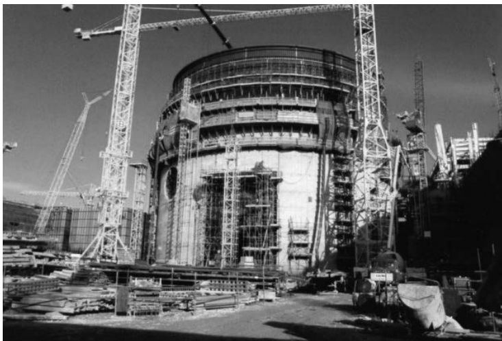
Fig. 3. Execution of Reactor Bldg. in Sizewell B power plant (photo by K. Tracz)
