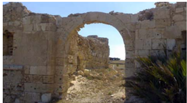
Fig. 30. Photo showing the entrance gate
