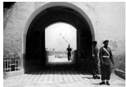
Fig. 25. The entrance gate; old photo dated 1975 in which military guards are there
