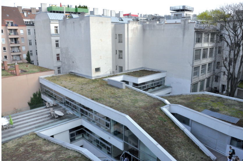
III. 7. Multifamily housing, Vienna, R. Delugan, E. Delugan-Meissl, 1999 (photo by P. Haupt, 2011)
