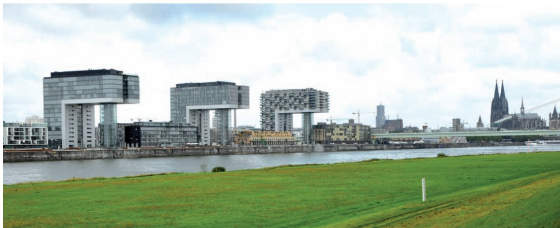
III. 1. Contemporary silhouette of Cologne – port district of Rheinauhafen with the characteristic buildings of Kranhäusern, Cathedral in the background (photo by K. Racoń-Leja)
