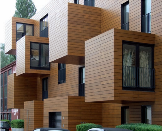
III. 18. Residential building WOHNRIEGEL BOGENALLEE – Hamburg. Housing architecture. “Flex boxen” bay windows (photo by W. Seruga)
