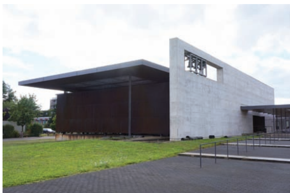
III. 23. Völklingen-Ludweiler, Parochial Centre of the Sacred Heart, designed by Lamott+Lamott Freie Architekten, 2001
