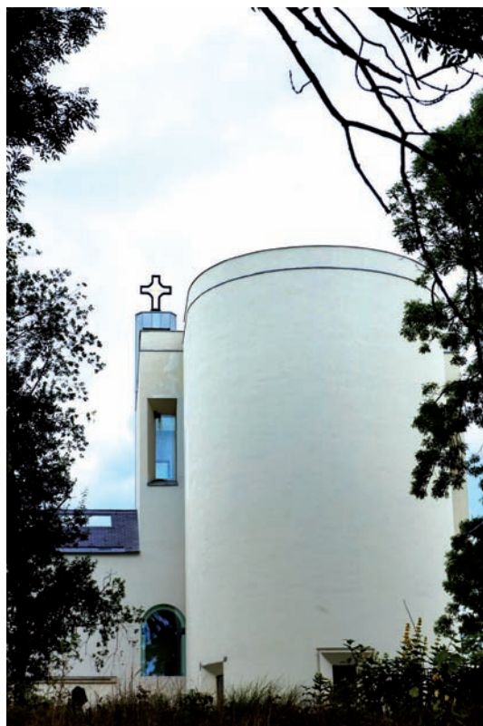
Ill. 7. Trappist Monastery in Nový Dvůr, extension, designed by J. Pawson, 2004
