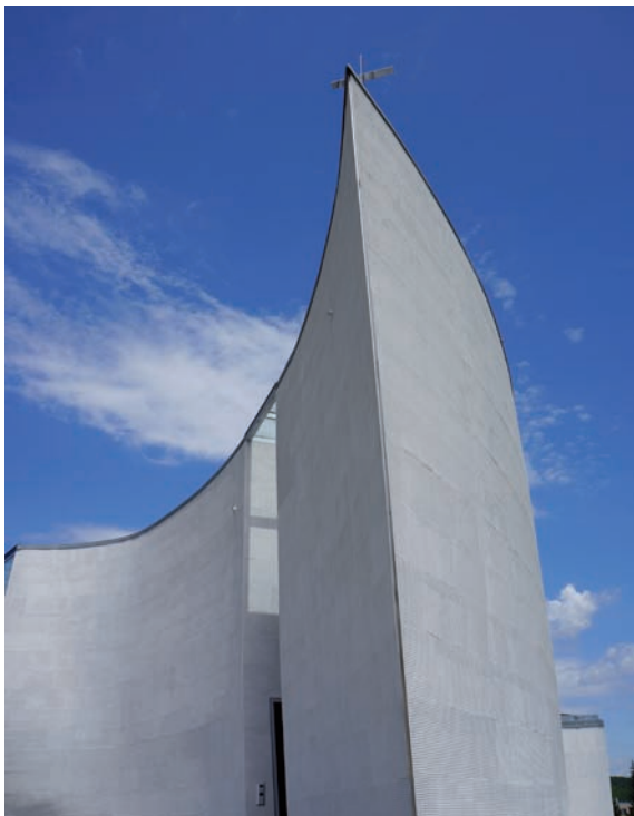
Ill. 19. Cernosice, new chapel, designed by Zdeněk Fránek Architects, 2010
