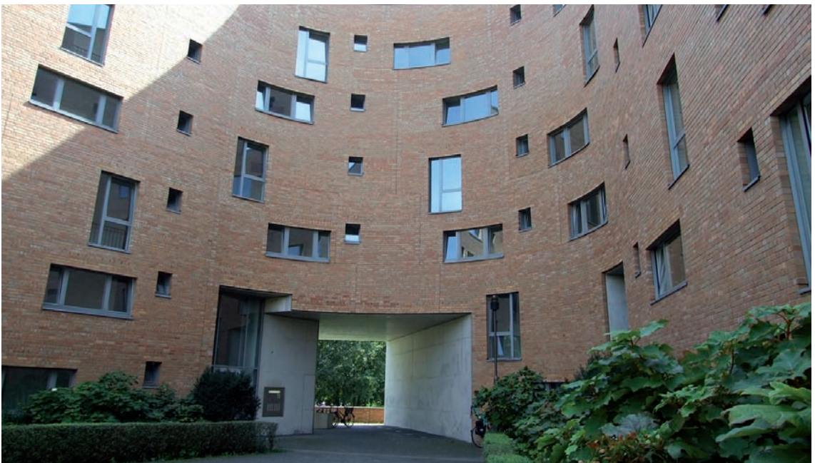
III. 2. Residential complex SNAKE – Berlin. Housing architecture. Pedestrian crossing connecting the northern urban enclosure with the southern urban enclosure (photo by W. Seruga)
