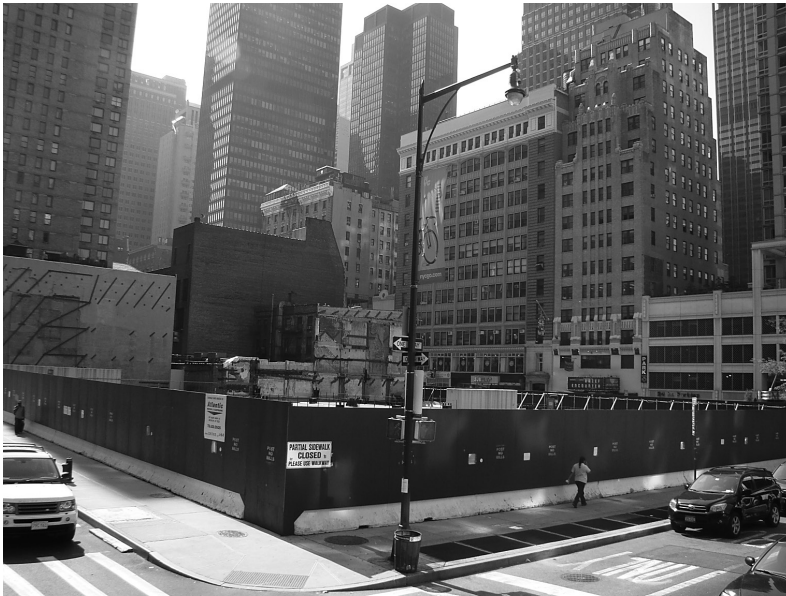
III. 21. View of the building site of a new apartment block on the corner 55th West St. and 8th Ave. in Manhattan. Previously the site had been occupied by traditional New York tenements (photo by D. Kuśnierz-Krupa, 2010)
