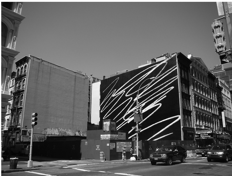
III. 22. View of the building site of a new apartment block on the corner of Howard St. and Broadway. Previously the site had been occupied by traditional New York tenements like the ones adjacent to the plot (photo by D. Kuśnierz-Krupa, 2010)
