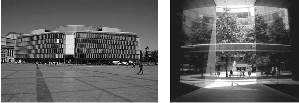
Ill. 3. Norman Foster, Metropolitan Building, Pilsudski Square, Warsaw, 1997–2003; a) View from Pilsudski Square, b) courtyard (photo by A. Szczepczyński)
