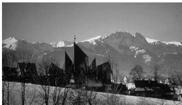
III. 17. Teresa and Tadeusz Gawłowski, Church at Olcza, Zakopane, 1978–1988 (photo by T. Gawłowski)
