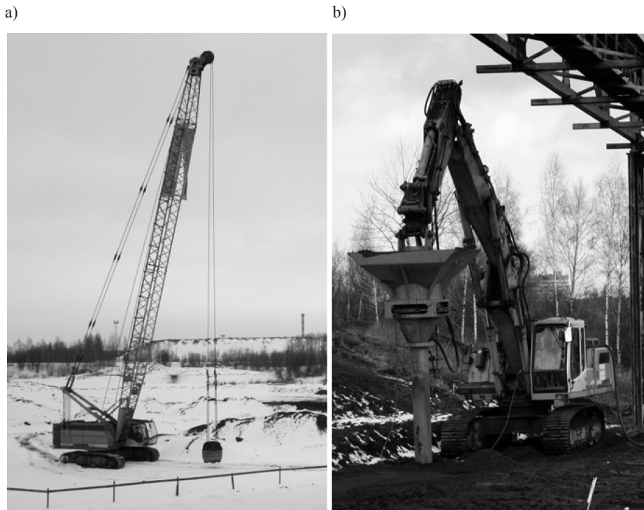
Fig. 1. Equipment for a) DR and b) VR column formation
