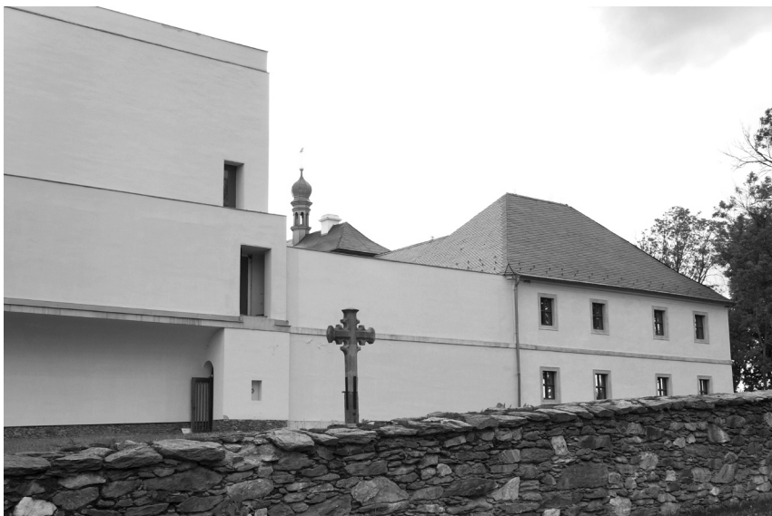
Ill. 6. Trappist Monastery in Nový Dvůr, extension, designed by J. Pawson, 2004
