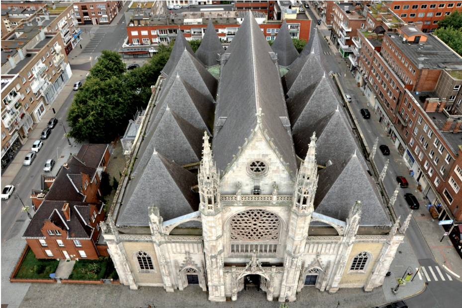
III. 5. 16 th century Saint-Eloi Cathedral in Dunkirk and the postwar surrounding buildings (photo by K. Racoń-Leja)
