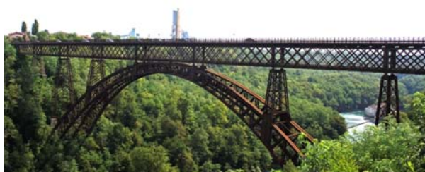
Fig. 1 Present up-stream view of the iron arch bridge (1889) from Paderno d'Adda (right bank)
