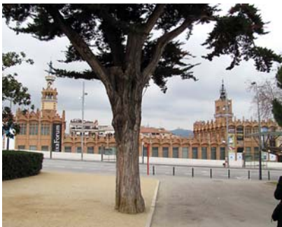
Ryc. 6. Widok ogólny Caixa Forum (dawnej fabryki Casaramona) z przeciwnej strony ulicy, spod pawilonu niemieckiego Miesa van der Rohe, fot. autor Fig. 6. General view of Caixa Forum (the former Casaramon factory) from the opposite side of the street, from the German pavillion by Mies van der Rohe – photo by author
