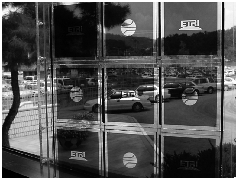
Fig. 2. Transparent DSC panel manufactured by ETRI and installed in one of its venues in Korea
