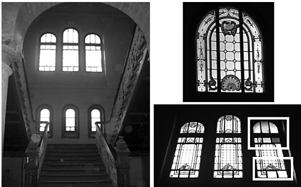
Fig. 17. Stair with remarkable stained glass used in windows, and its current status
