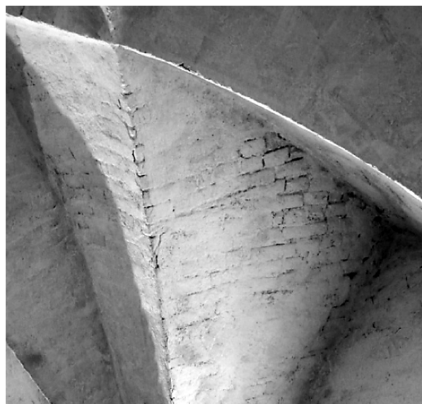
Fig. 5. Corrections in the direction of the courses carried out ad hoc by cutting bricks, indicate that the vault was constructed without formwork (D. Wendland)
