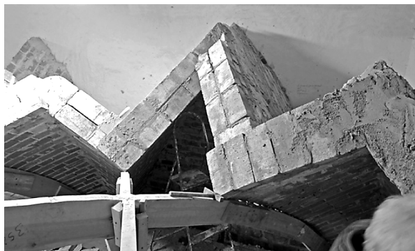
Fig. 13. Also in the higher portions the continuity over the whole squinch can easily maintained. Over the transversal cap, the courses are seamed (D. Wendland)
