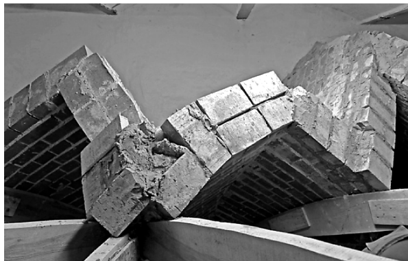
Fig. 14. At the intersection points in the groins, the direction of the masonry courses change. Never-theless, the continuity of the texture is maintained (D. Wendland)
