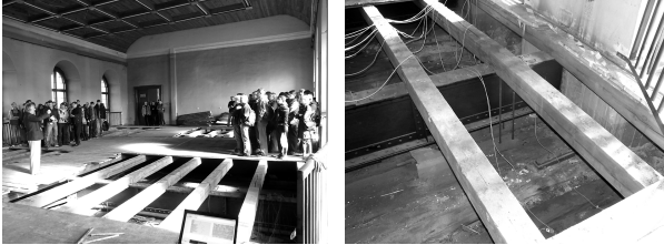
Fig. 16. View of the Balzer Hall above the Aula Leopoldina. Placement of measuring points in the Balzer Hall is shown in (Fig. 17) and model OMA in (Fig. 18).
