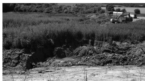
Fig. 4. Sediment removal by dredging
