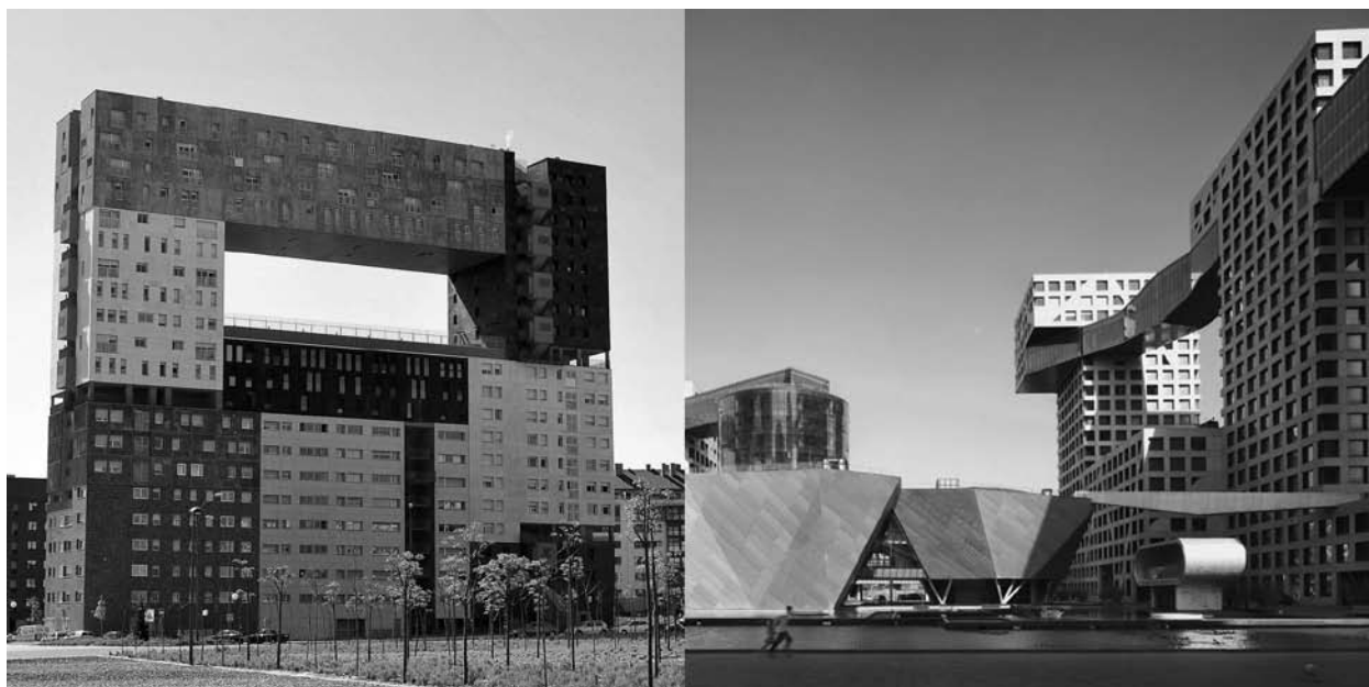
Mirador; Hybrid Building
