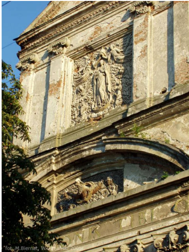
Rys. 3. Górny ryzalit fasady – fragment (fot. M. Biernat) Fig. 3. The part of the upper part of the façade (photo by M. Biernat)
