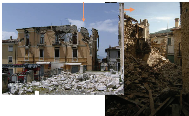
Fig. 3. Problems caused by the irregular and pushing roof timber systems
