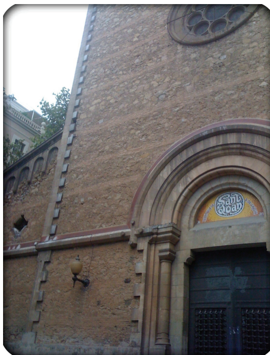
Fig. 14. "banded masonry" in the façade of Saint Joan church in Barcelona
