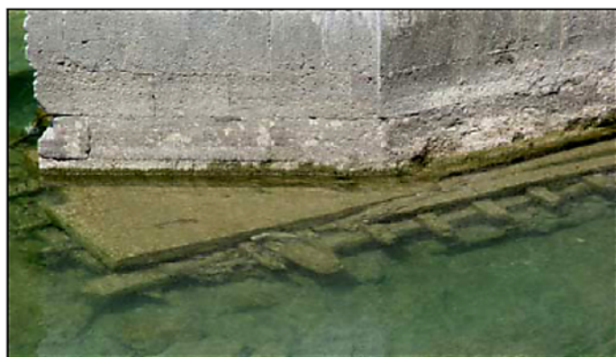
Fig. 7. Round wood foundation base of Konjic Bridge [6]
