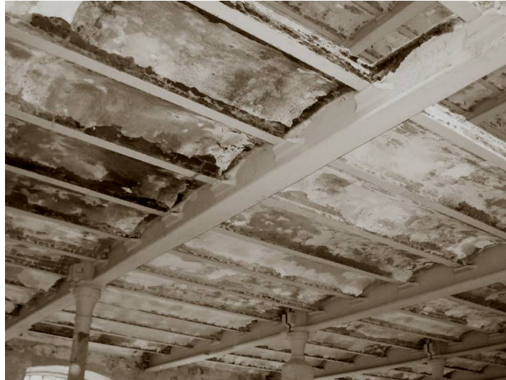
Rys. 3. Widok stropu Fig. 3. View of the floor
