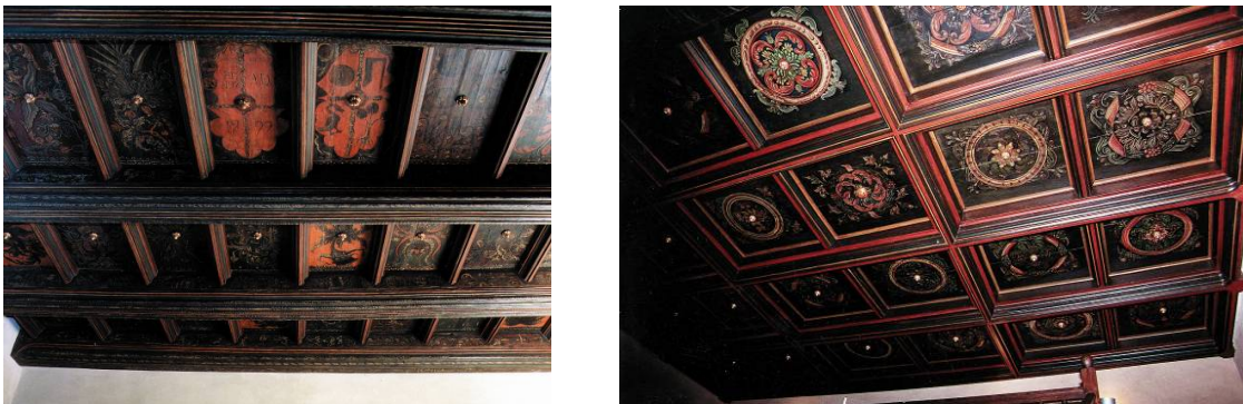
Rys. 8. Odrestaurowane stropy drewniane I piętro i parter Fig. 8. Renovated old wooden floors (first floor and ground floor)
