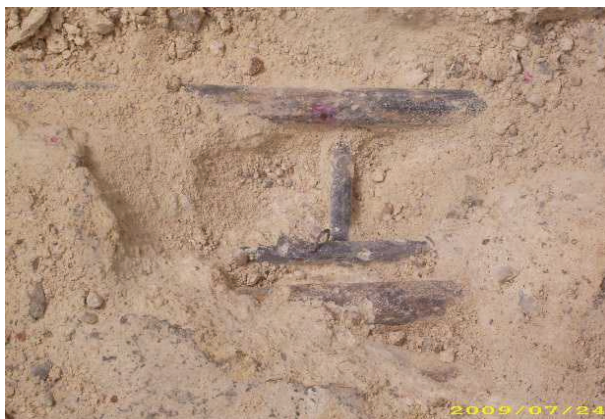
Rys. 10. Zbrojenie dna niecki basenu Fig. 10. Reinforcement in pool basin bottom
