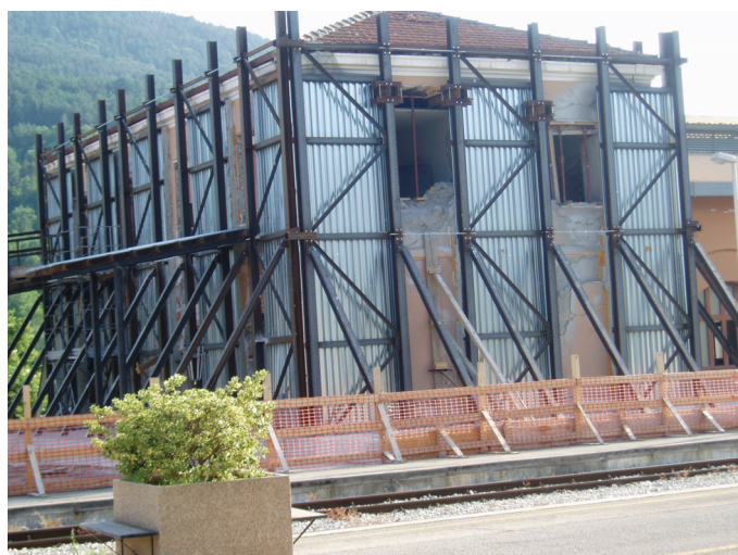
Fig. 9. Steel cage system with spur aid Rys. 9. System klatkowy
