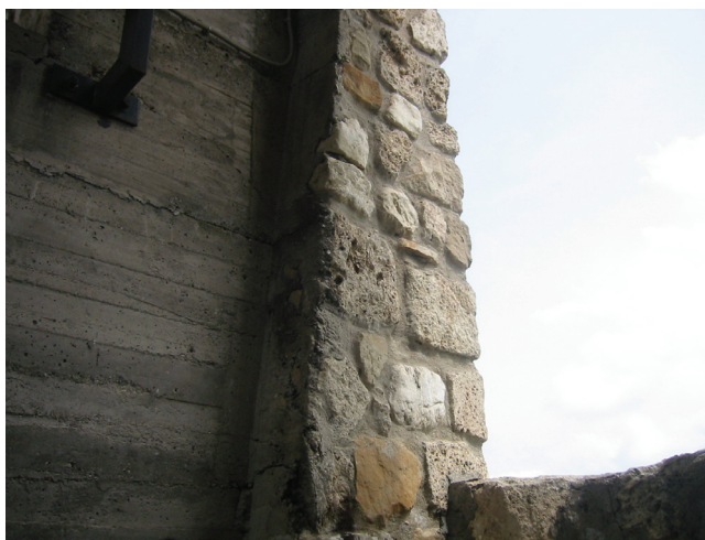
Fig. 12. Strong intervention using reinforced concrete and "false" masonry
