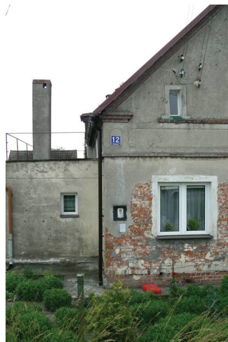
Rys. 6. Monitorowany stary budynek Fig. 6. Monitored old building
