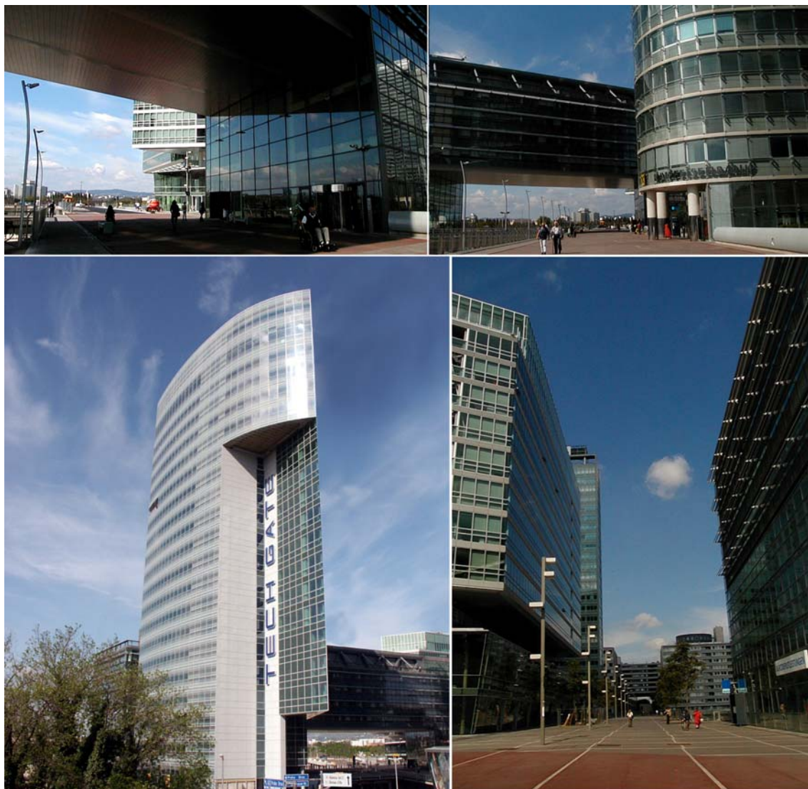
II. 1. Donau City, Tech Gate, photo. aut.
