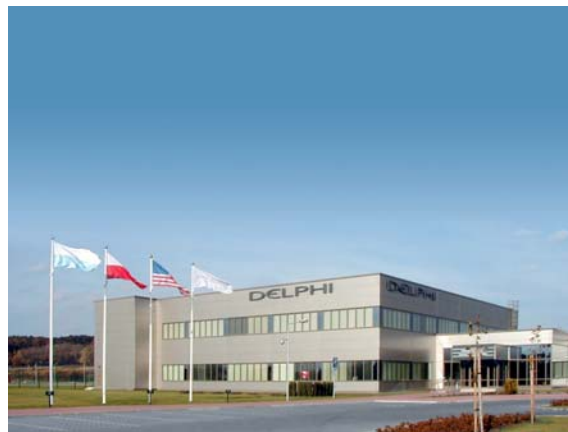
Fig. 1. View on Technical Center Kraków, Delphi SA Poland Rys. 1. Widok Centrum Technicznego Kraków, Delphi SA Poland
