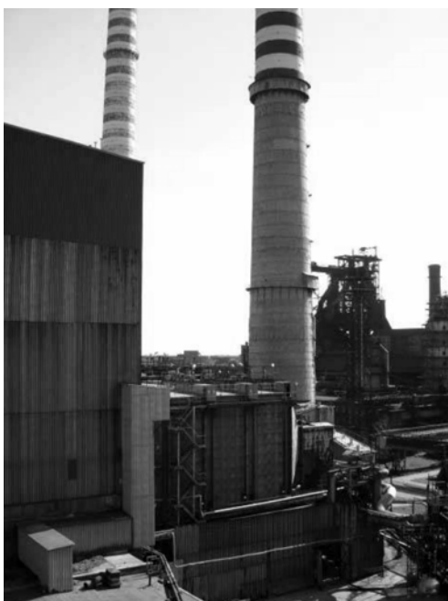
Fig. 2. General view of the ArcelorMittal Steel Poland Power Plant in Kraków
