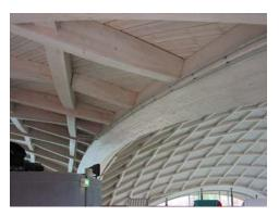
Fig. 9, 10. Toscana Therme Bad Sulza, Germany. Interior – curved roof-shell with the grating-structure. Photo S. Kuc
