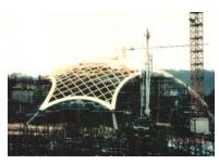
Fig. 7. Toscana Therme Bad Sulza, Germany. Shell structure in wood-grating. Photo O. Büttner
