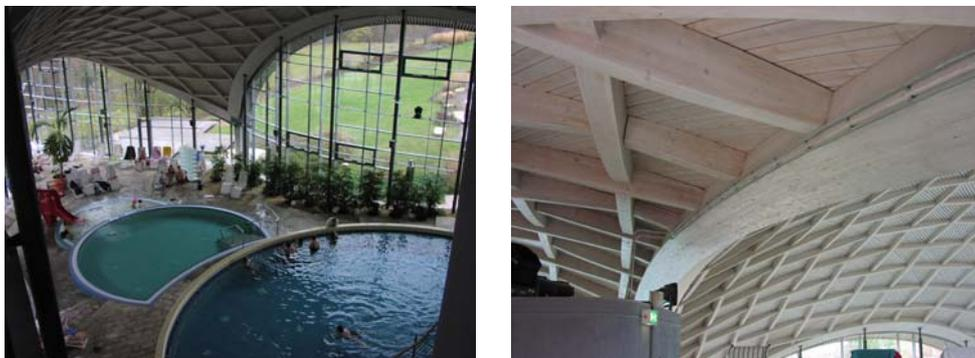
Fig. 9, 10. Toscana Therme Bad Sulza, Germany. Interior – curved roof-shell with the grating-structure. Photo S. Kuc
