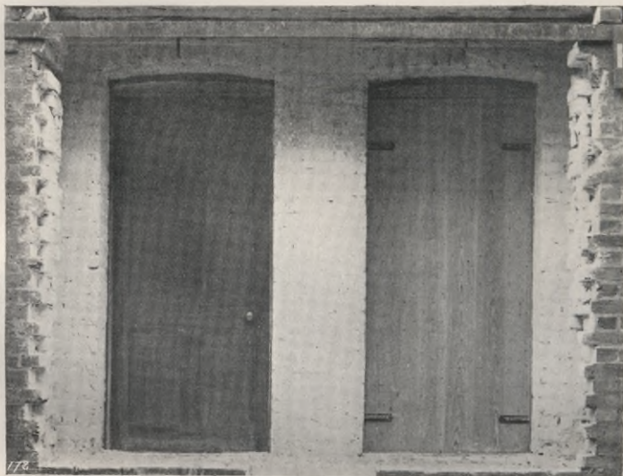
Fig. G. VIEW OF DOORS BEFORE TEST (FROM OUTSIDE).
