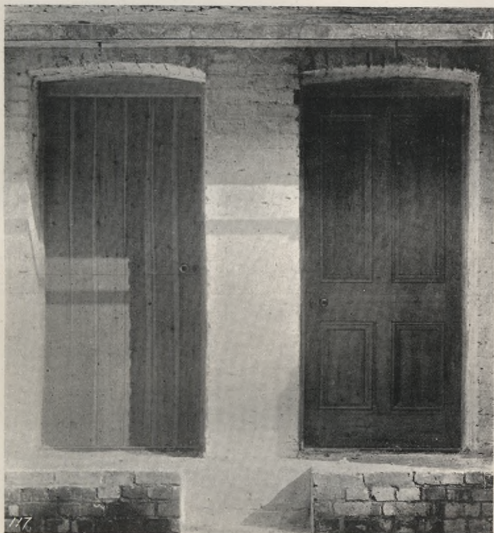
THE DOORS. Fig. G. VIEW BEFORE TEST (FROM OUTSIDE).
