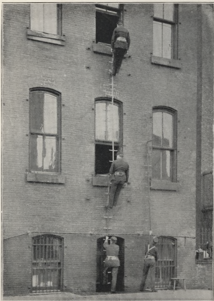
SCALING LADDERS, AS USED AT NEW YORK.
