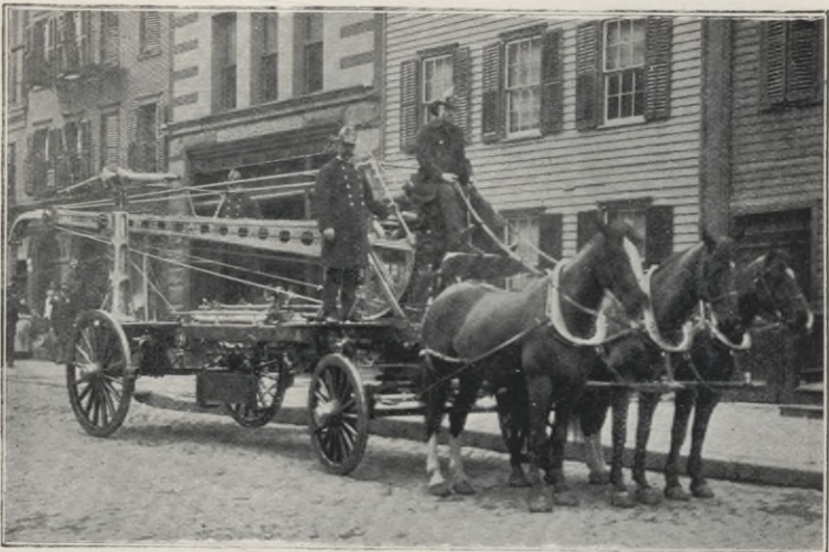
THE WATER TOWER, LOWERED FOR MOVEMENT THROUGH THE STREETS.
