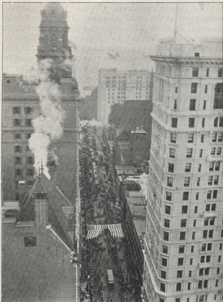
FIG. 11. SUGGESTIVE OF THE DIFFICULTY OF REACHING THE UPPER STORIES OF A SKY SCRAPER WITH A FIRE STREAM.
