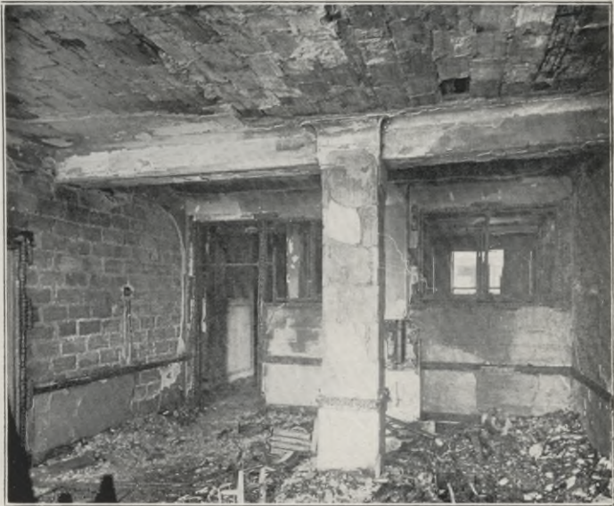
FIG. 6. 10TH FLOOR. COLUMN AND GIRDER COVERINGS AND PARTITIONS INTACT.
