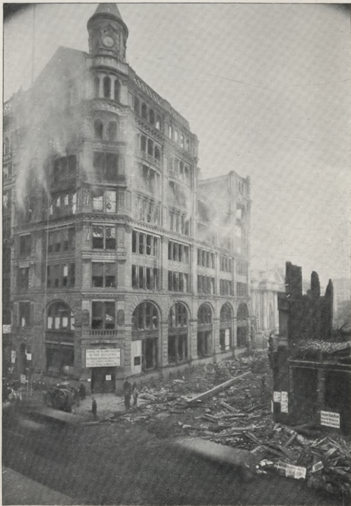
FIG. 3. A FIRE-PROOF BUILDING WRECKED BY A FIRE ACROSS THE STREET.
