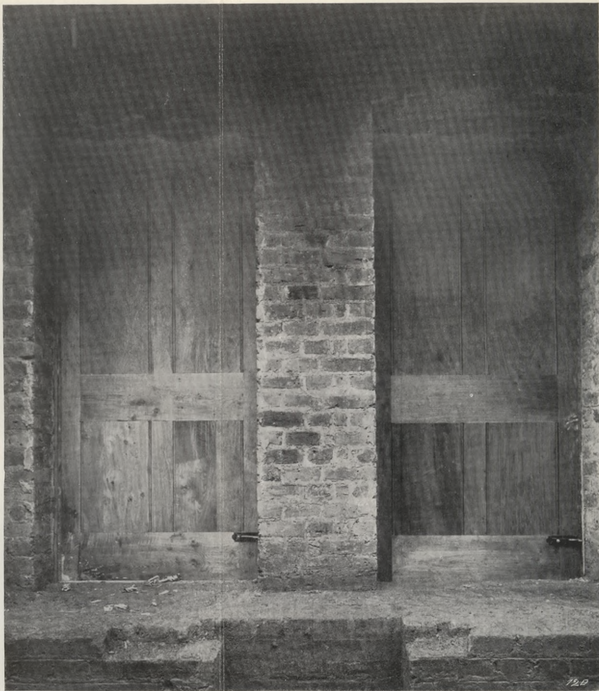
Fig. G. VIEW OF DOORS BEFORE TEST (FROM OUTSIDE).
