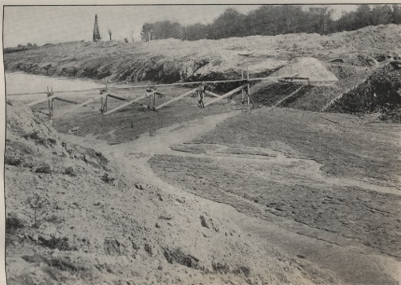
BARGE CANAL, CONTRACT No. 44.
