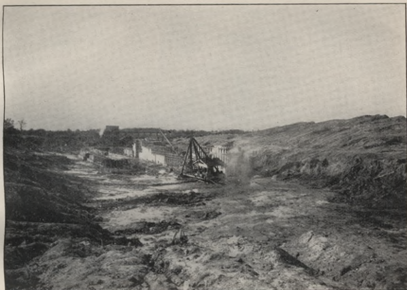
BARGE CANAL, CONTRACT No. 44.
