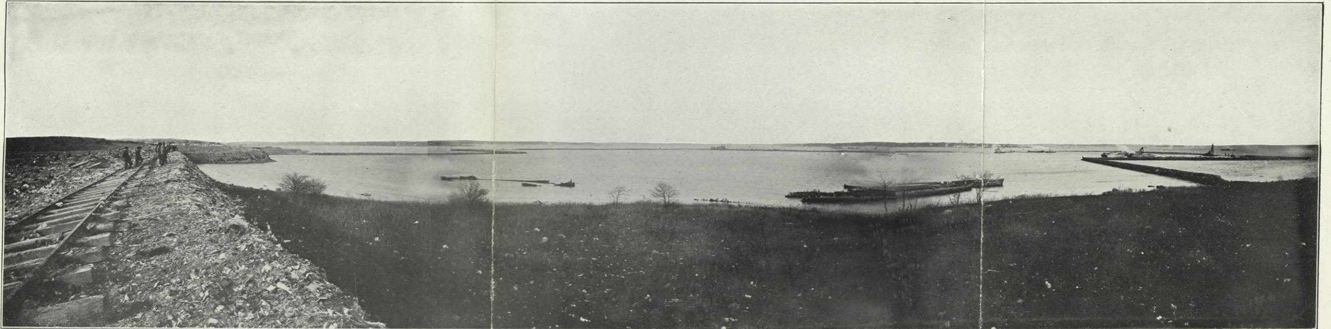
BASIN OF 147 ACRES AT RIKERS ISLAND CREATED BY THE CONSTRUCTION OF 1.7 MILES OF BULKHEAD OR RETAINING WALL, TO BE FILLED IN BY REFUSE FROM THE DEPARTMENT OF STREET CLEANING
