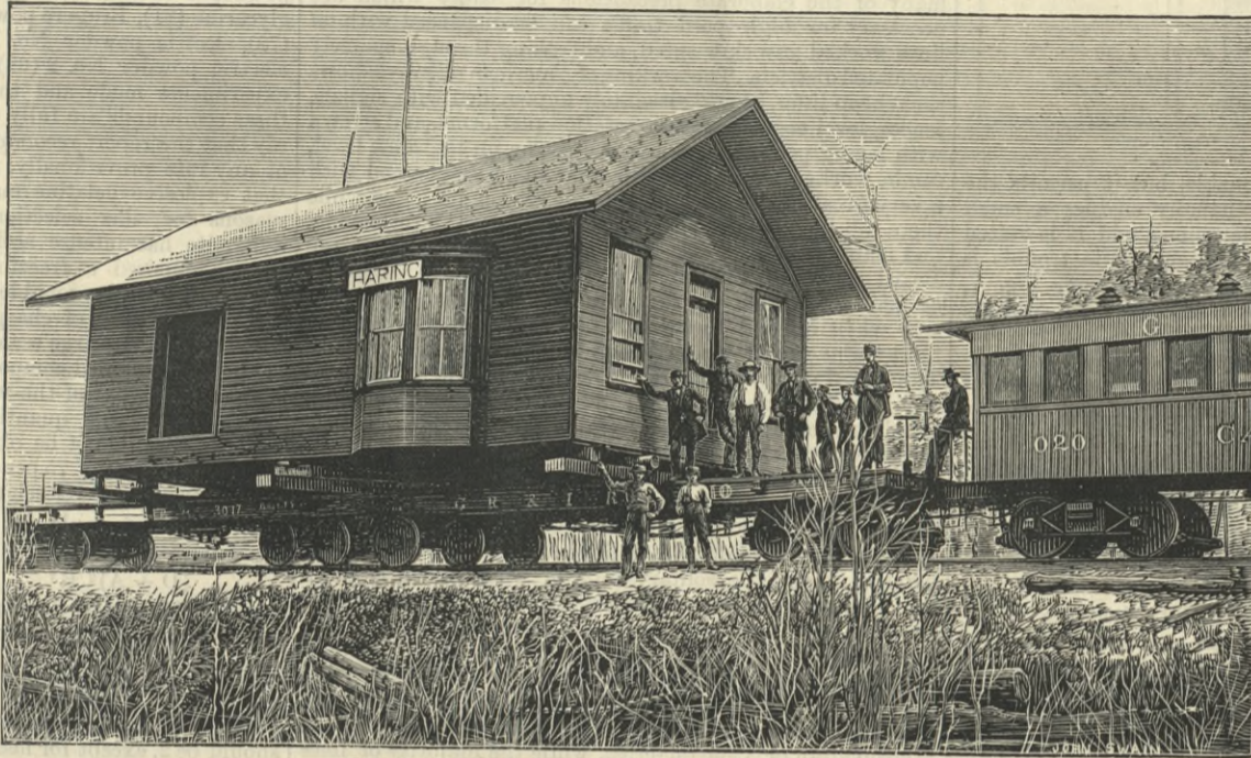
FIG. 9.—MOVING AN AMERICAN RAILWAY STATION.
