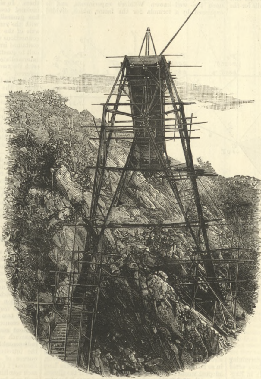
BRIDGE IN PROCESS OF ERECTION
