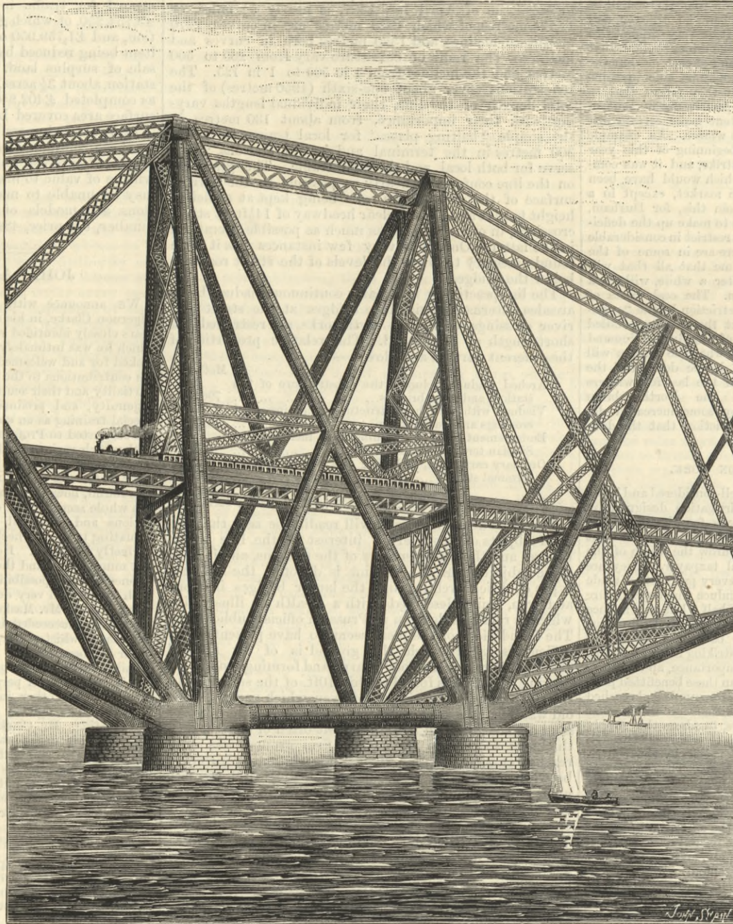
Fig. 2—A MAIN CANTILEVER PIER.
