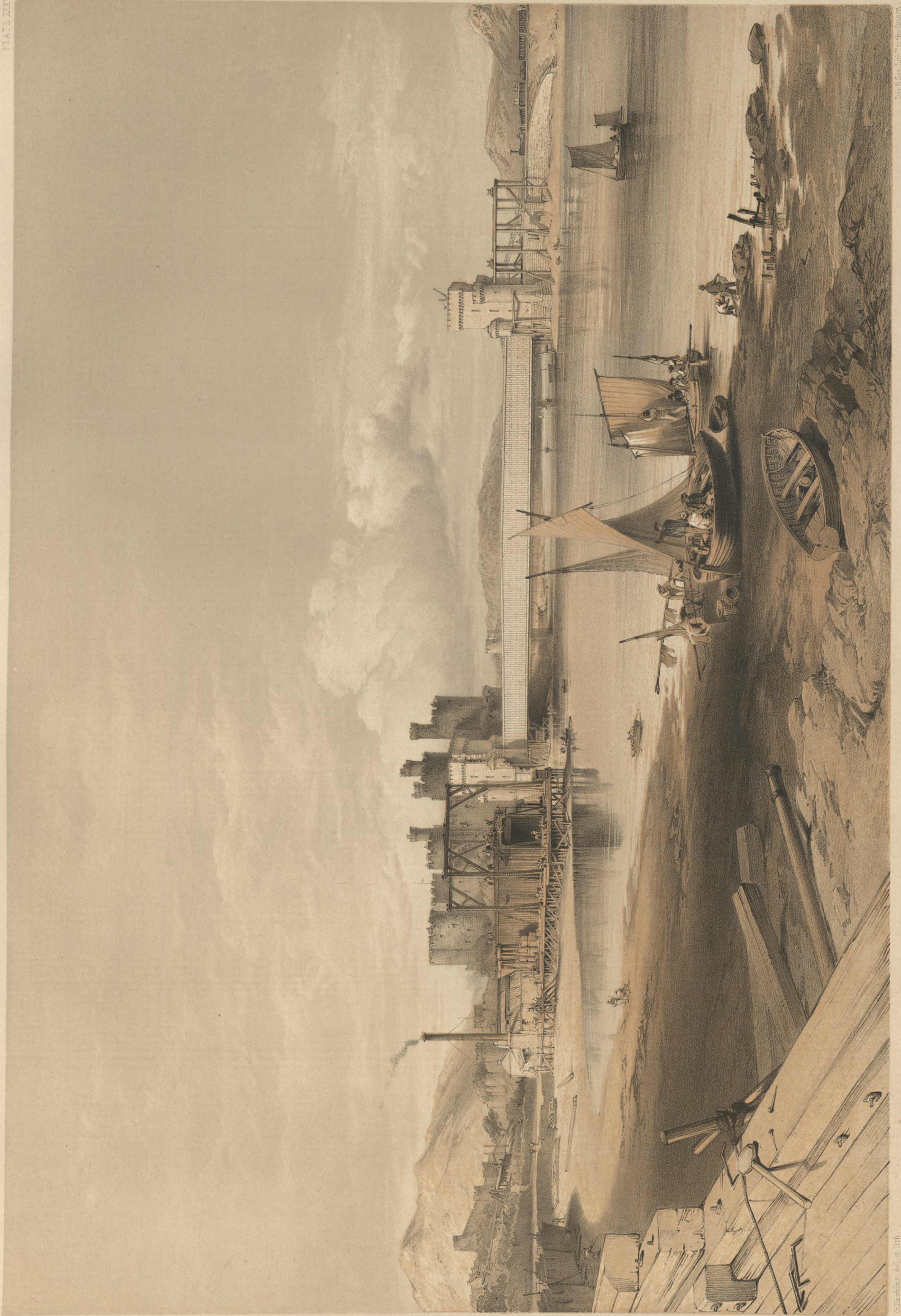
CONWAY BRIDGE. CONSTRUCTION OF SECOND TUBE, SEPTEMBER, 1848.
