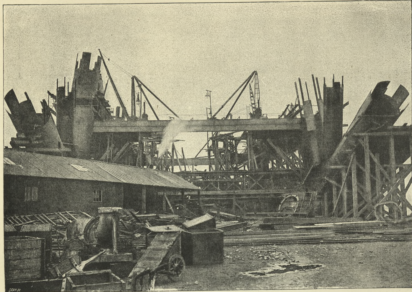
FIFE PIER. ERECTION OF SUPERSTRUCTURE ; CONSTRUCTION OF LIFTING PLATFORMS.
