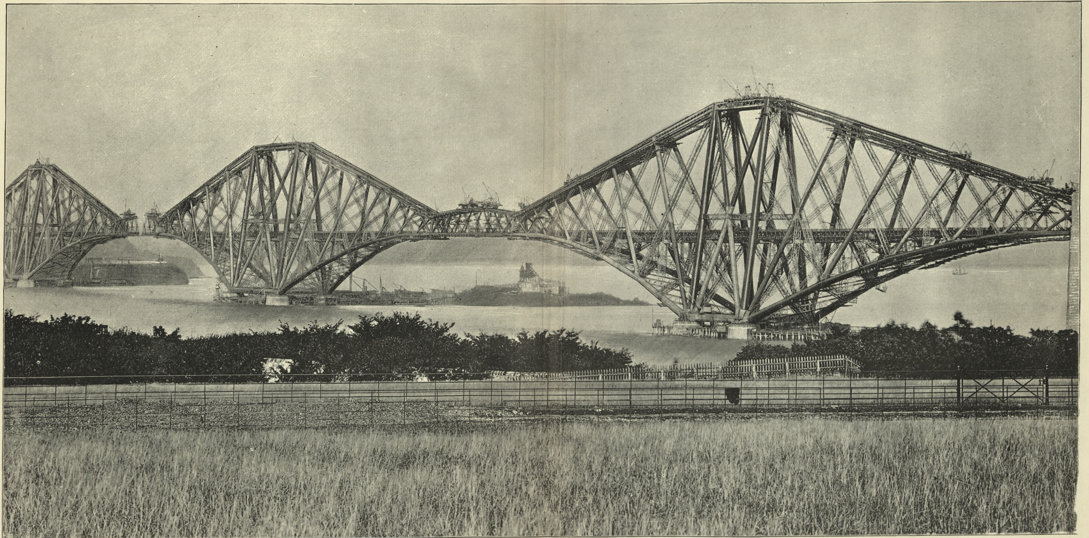
GENERAL VIEW OF BRIDGE. SOUTH CENTRAL GIRDER CONNECTED—NORTH CENTRAL GIRDER NOT COMPLETED.
