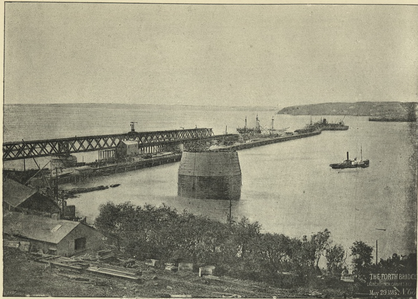
LAUNCHING OF CAISSON FOR SOUTH-WEST PIER, INCHGARVIE.
