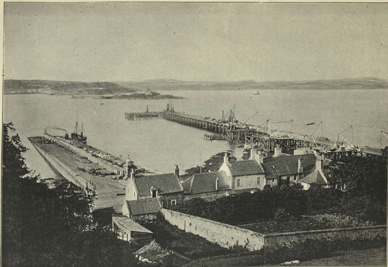
GENERAL VIEW OF SITE LOOKING NORTH-EAST.
