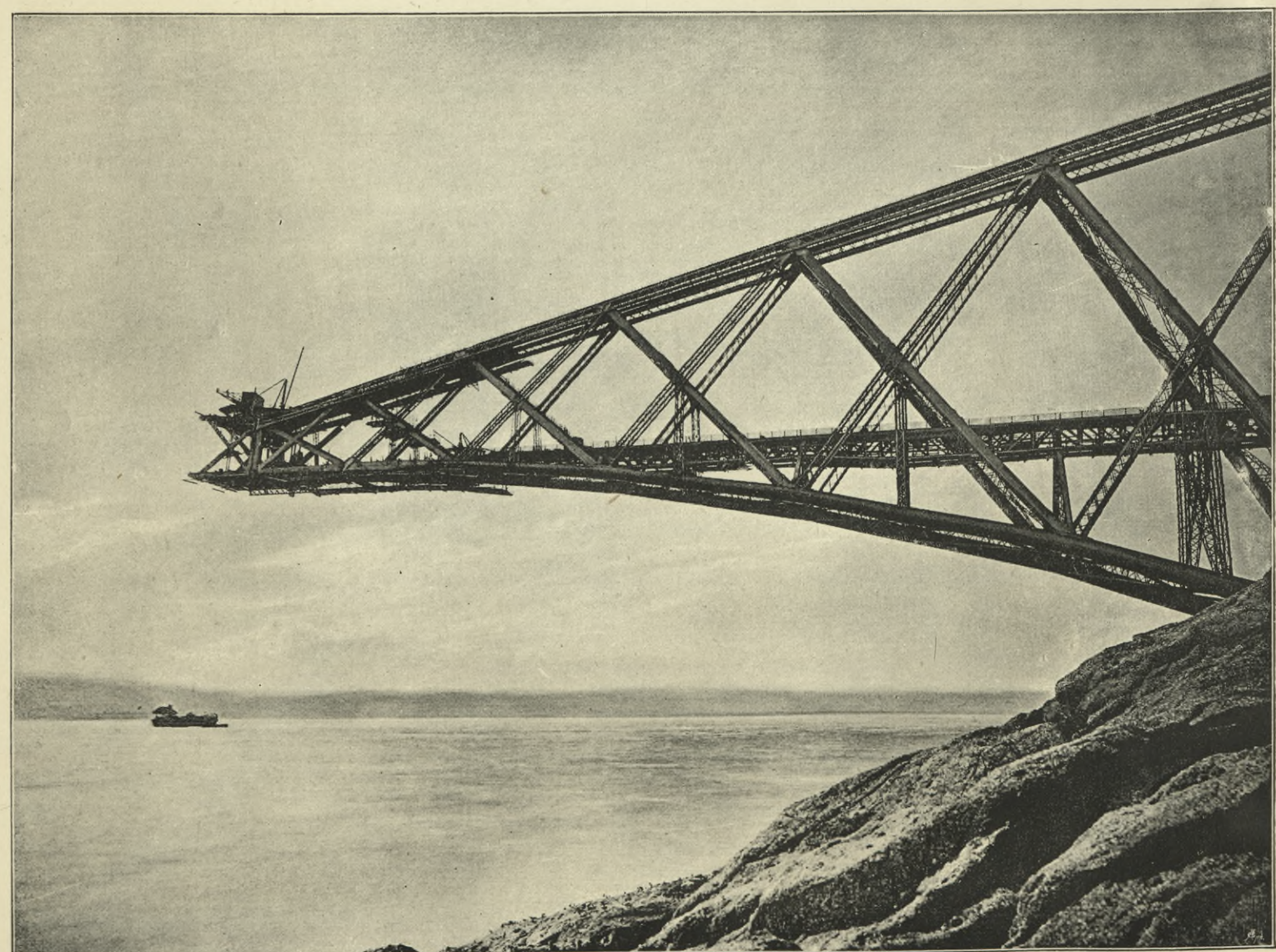
INCHGARVIE SOUTH CANTILEVER, WITH FIRST BAY OF CENTRAL GIRDER BUILT OUT.
