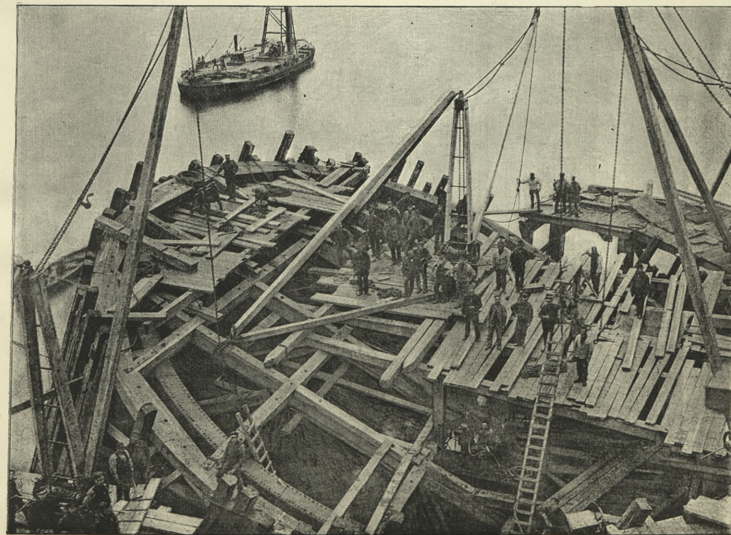
CAISSON FOR QUEENSFERRY NORTH-WEST PIER. CONSTRUCTING TIMBER CASING ROUND THE TILTED CAISSON.
