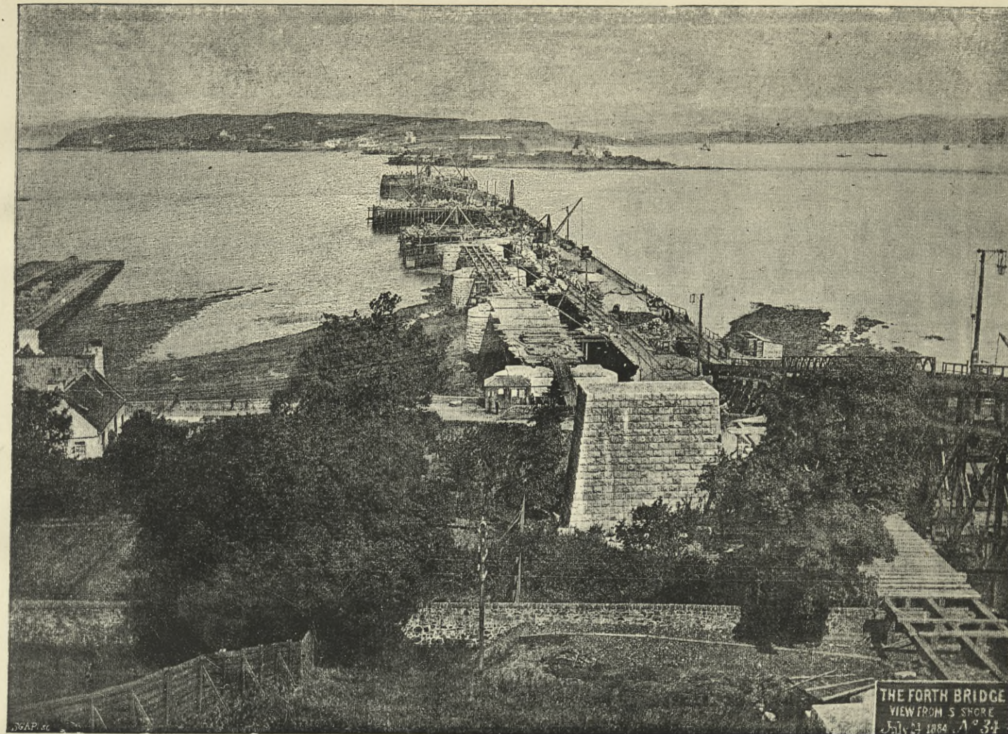
GENERAL VIEW OF SITE, WITH PIERS OF SOUTH APPROACH VIADUCT, LOOKING NORTH.
