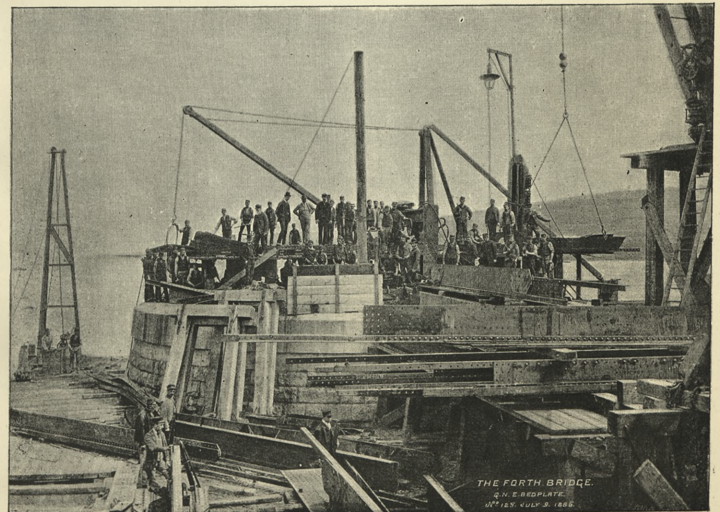
QUEENSFERRY NORTH-EAST PIER. PUTTING TOGETHER UPPER BEDPLATE.
