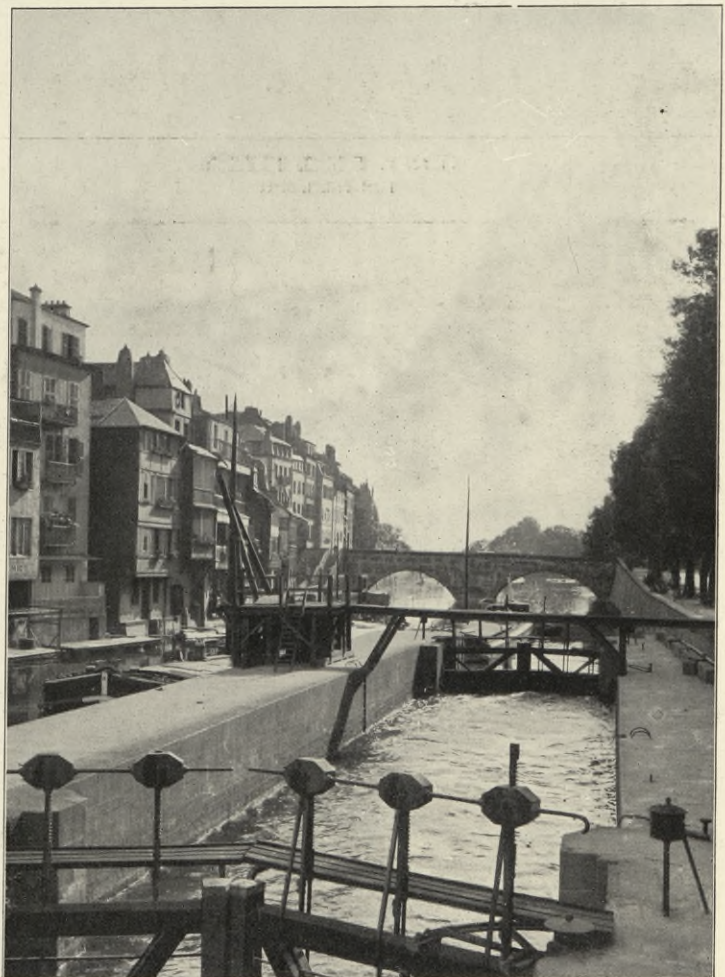
Metz. Schleuse Phot. Prillot, Metz
