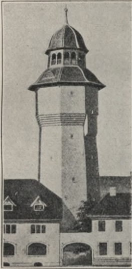
Abb. 100. Wasserturm in Nyköping.
