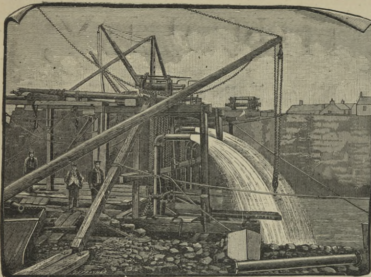
Pulsometers raising 340,000 gallons per hour from a Caisson.
