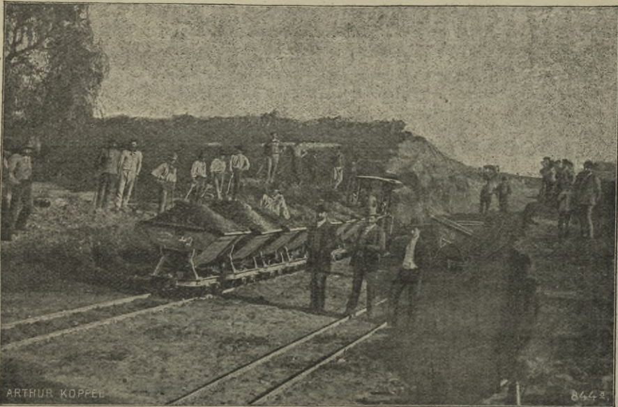
EXCAVATION WORK IN THE ARGENTINE.
