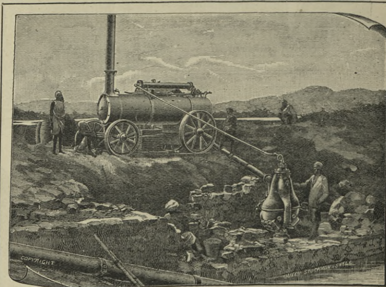
Illustration is from Photo. of an Irrigation job in India carried out by means of a Pulsometer.
