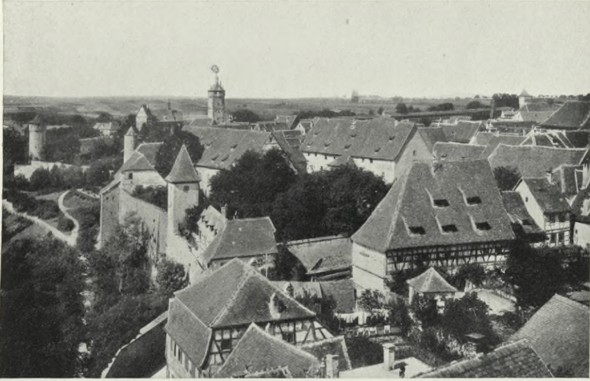
Illus. 105.—Rothenburg, Standpoint VI. on Fold Plan III., showing the country coming right up to the town.
