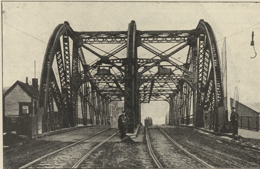
Archer-Avenue-Brücke in Chicago. Fig. 150.
