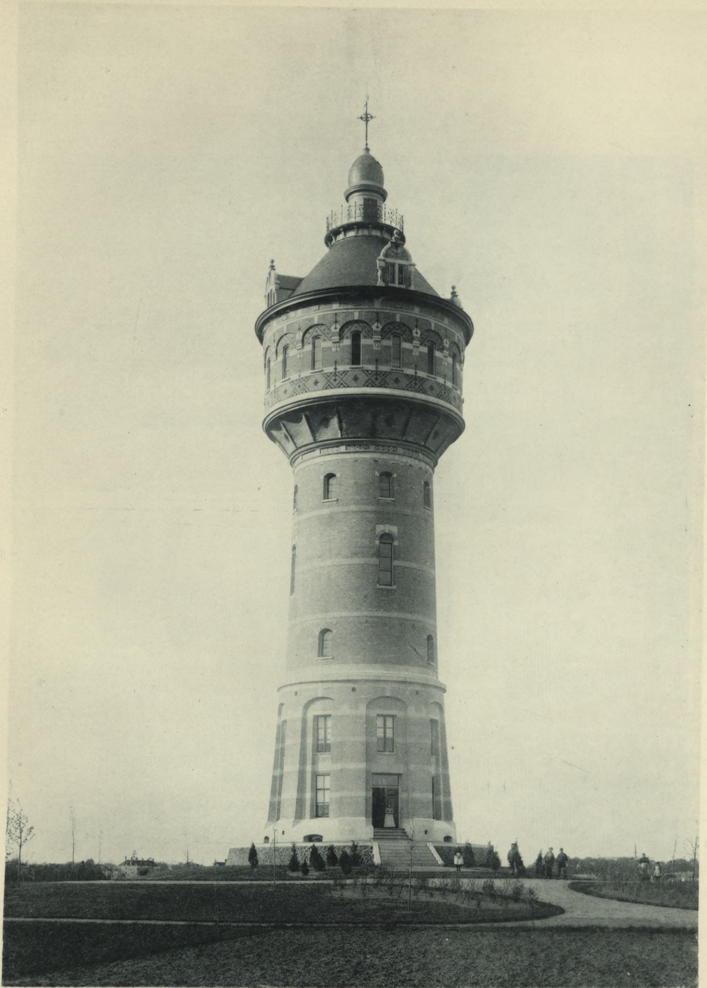
Wasserthurm Deventer (Holland), 500 cbm. Ingenieur Moulock Houwer in Deventer.
