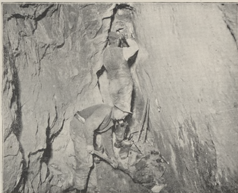
Fig. 43. Miners at the preliminary work of tracing the course of a vein of metal-bearing ore.
