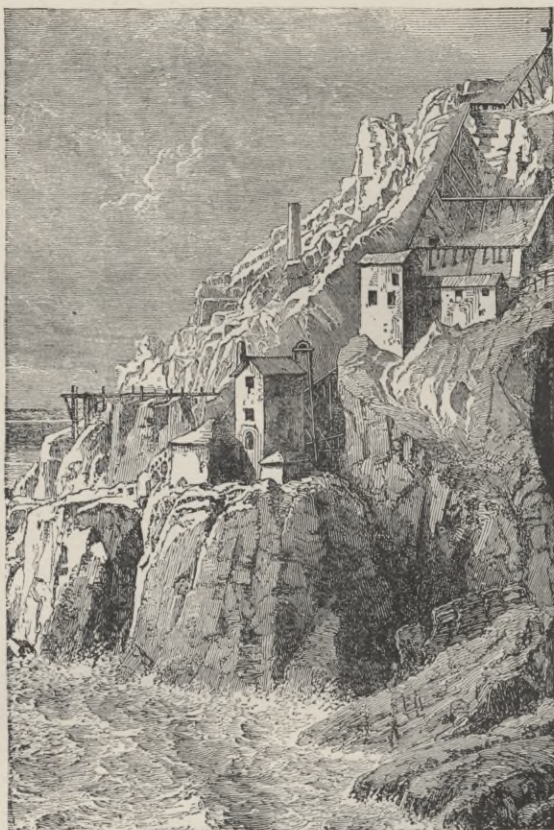
Fig. 69. Surface works of Botallack tin mine, Cornwall, England. (The shafts are 1,050 feet deep; the horizontal levels stretch 1,200 feet under the sea.)
