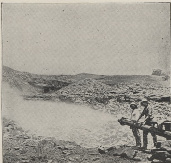
Fig. 56. Washing auriferous earth by the hydraulic method (South Africa).
