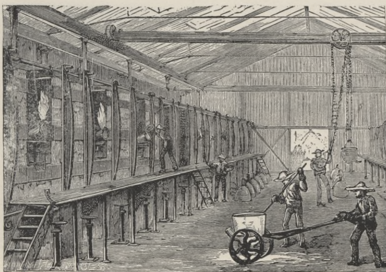
Fig. 5. Exterior view of Castner sodium furnaces.
