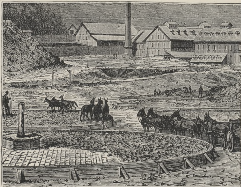
Fig. 35. Mexican patio. A mixture of silver ore, salt, sulphates, and mercury, trodden by mules leads to a decomposition of the ore and to an absorption of the silver by the mercury.
