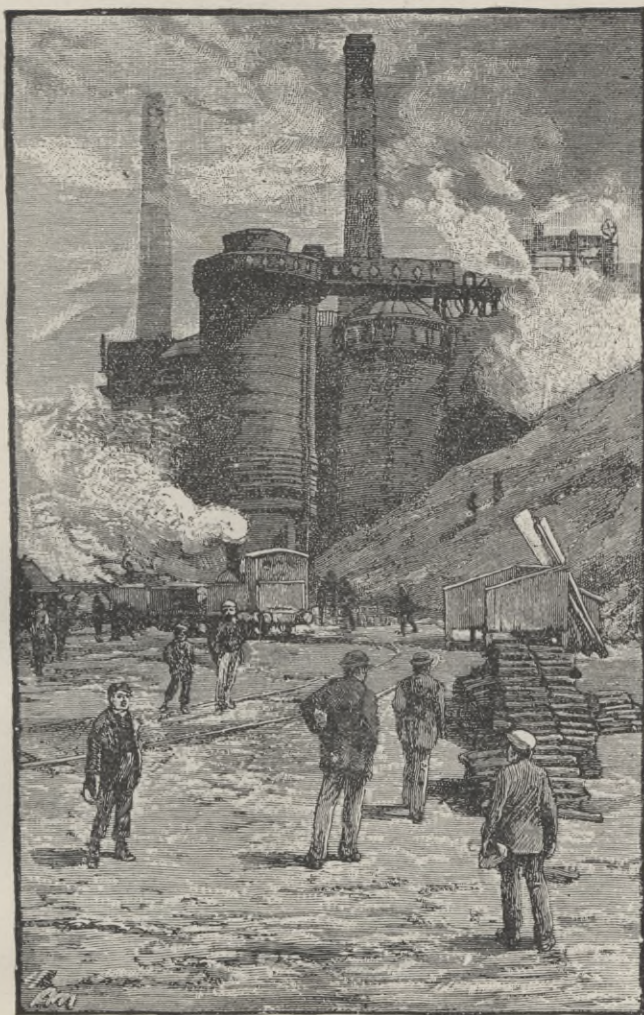
Fig. 85. English blast furnace for production of pig iron.
