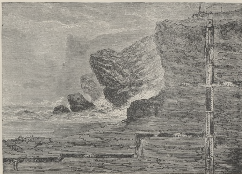
Fig. 70. Subterranean shafts and galleries of Botallack tin mine, Cornwall, England.
