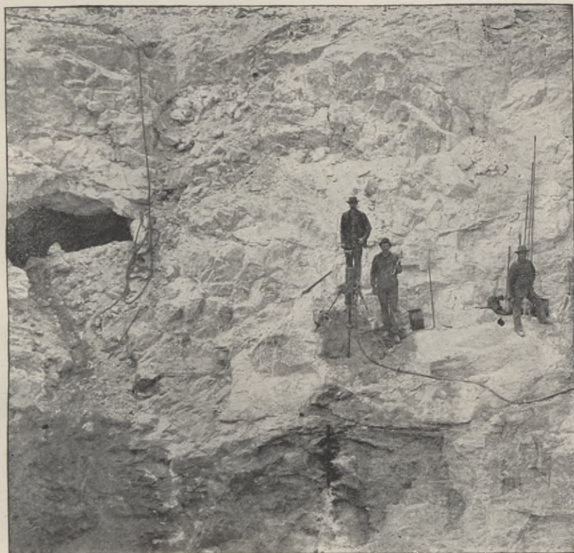
Fig. 54. In the pit—Alaska-Treadwell mine, near Juneau, Alaska. The men are drilling the rock preparatory to blasting.
