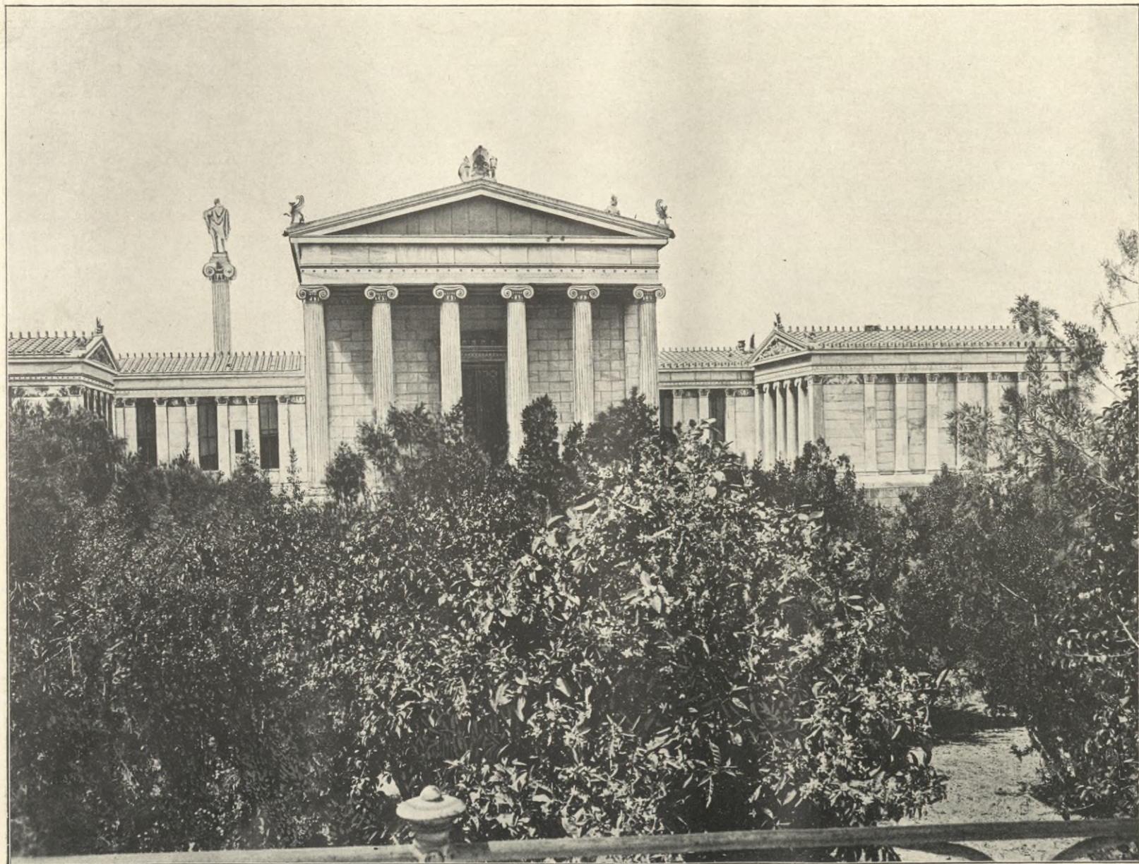
Rear View of Academy Building
