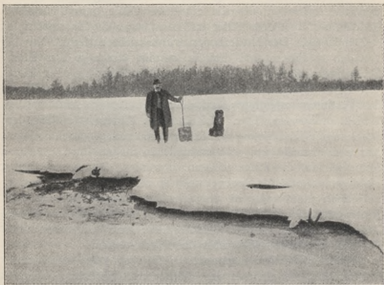
Fig. 84. Intermittierendes Filter in Framingham zur Winterszeit.
