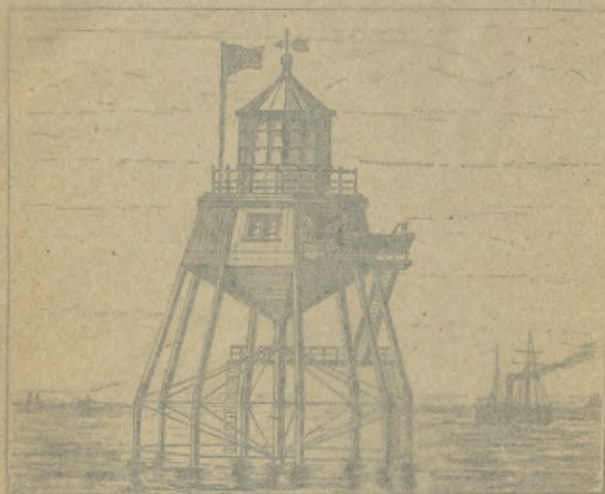
Maplin Screw Pile Lighthouse.
